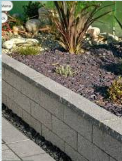
花槽配設花崗岩牆壁 Granite walls around planting beds in performance area
