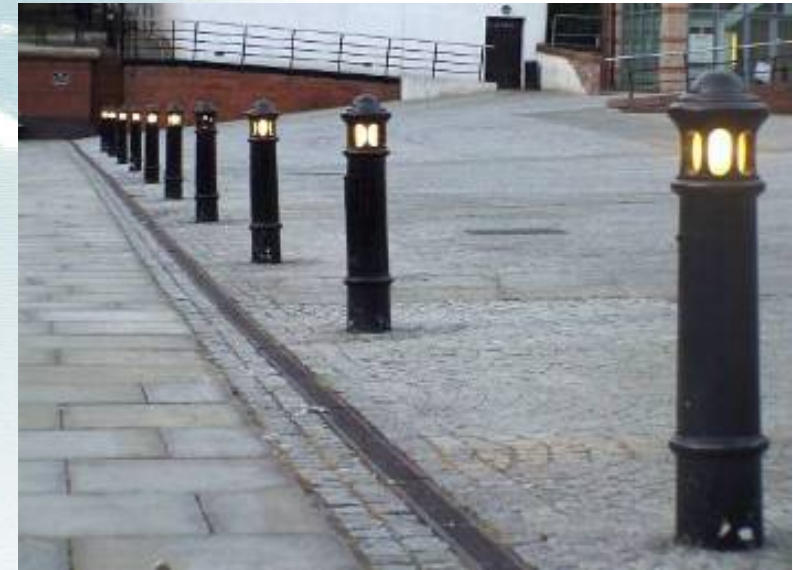
路邊燈柱 Road-side bollards
