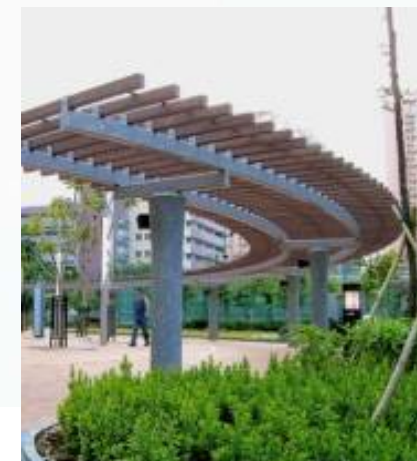
有蓋行人道 Covered walkway
