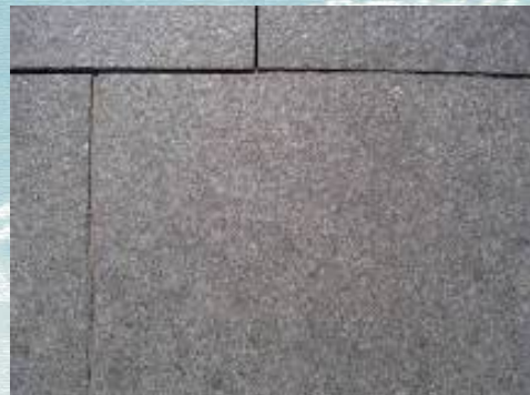
高質素地磚 High quality paving
